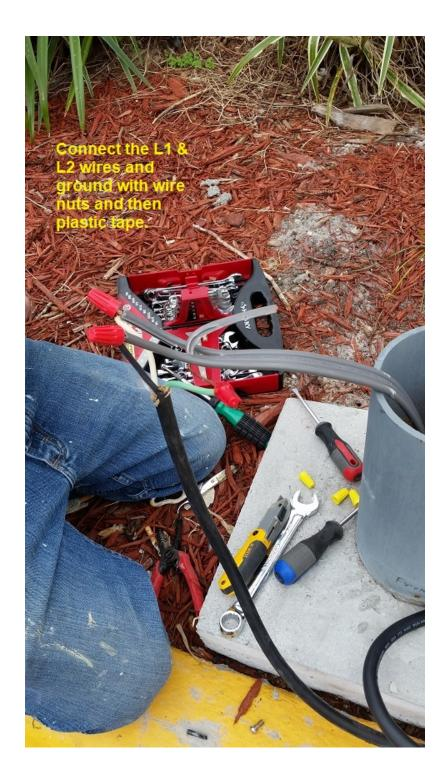
Install on a concrete 12" square by 4-6 inch thick pad.
